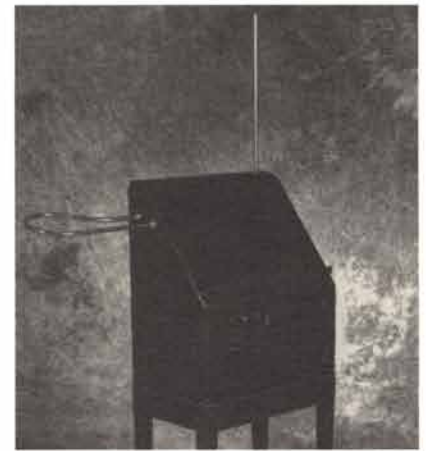
The Theremin, manufactured by RCA, ca 1931 (710502)
